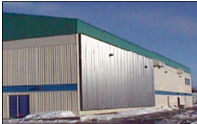
Figure 4 - Photo of grey SolarWall panels on wall of gym
