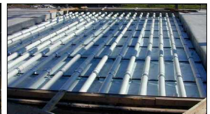
The excess heat taken off the solar panels is ducted into the concrete radiant in-floor heat storage system, shown left after completion, and shown above during installation.
