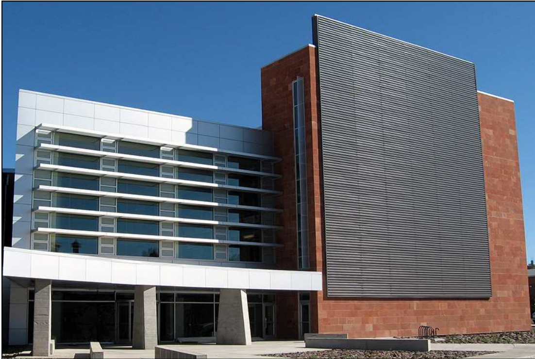
Charcoal SolarWall® air heating system installed at Northern Arizona University's new LEED® Silver Distance Learning Center.
