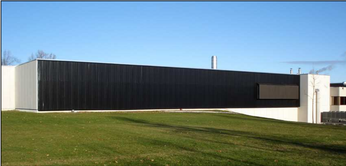
Left, the completed SolarWall® solar air heating system at MDS Nordion's Ottawa location on the southwest facing wall
