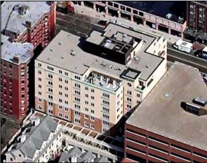
The SolarWall® solar air heating system is located on the penthouse of Houghton Place Apartments
