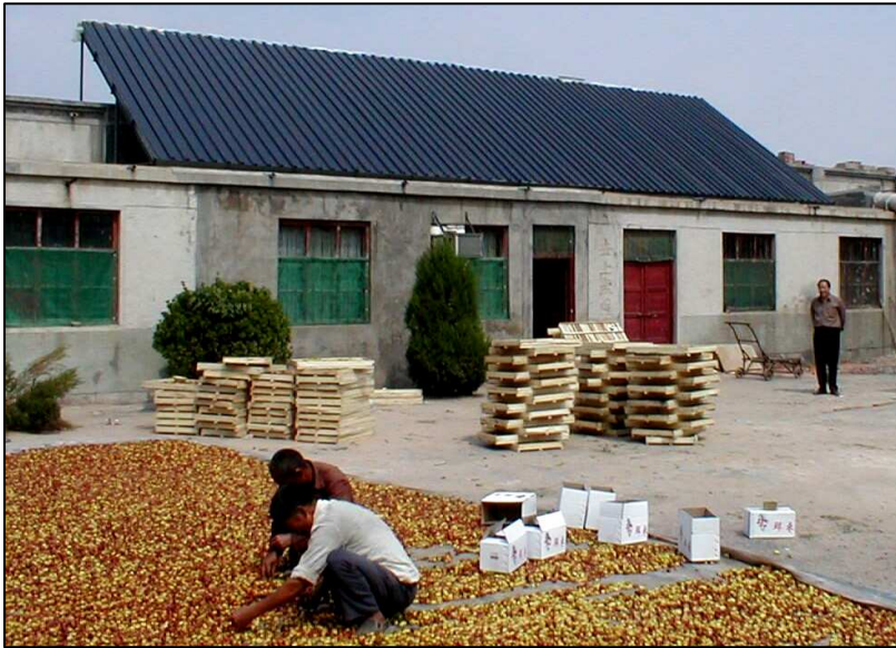
600 ft 2 of roof mounted SolarWall ® panels provide heat to the fruit dryer.
