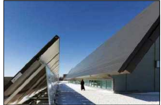
The grey SolarWall® system on CANMET's Materials Technology Laboratory at Hamilton's McMaster Innovation Park—at a 53 degree angle on the south façade of the new facility
