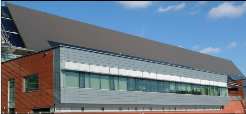
The grey SolarWall® system on CANMET's Materials Technology Laboratory at Hamilton's McMaster Innovation Park—at a 53 degree angle on the south façade of the new facility
