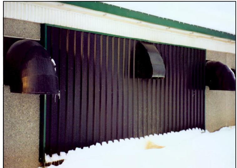
SolarWall® system preheating air to heat recovery ventilator
